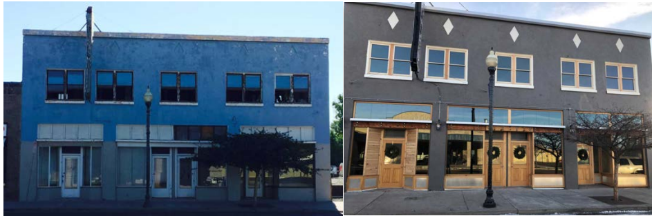
Central Hotel, Burns 2017 awarded project. Vacant for 40 years and now a hotel and two businesses.
