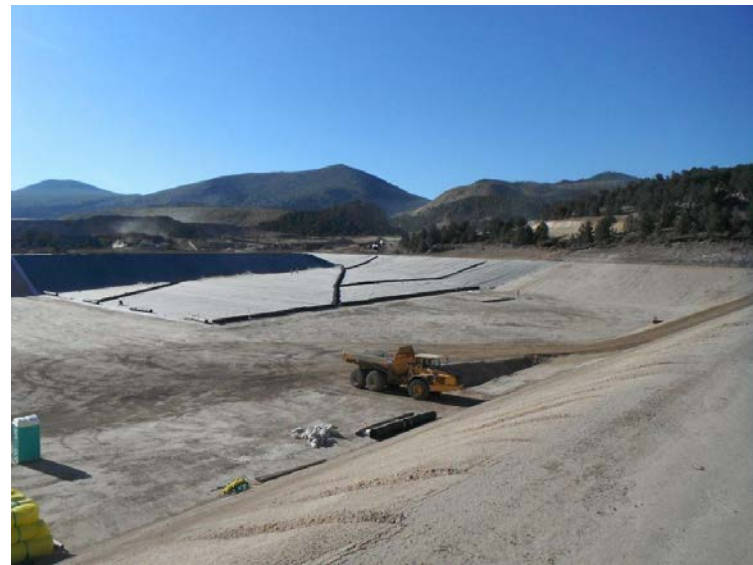
Esmeralda Mill, Nevada, 100 acres, rubber-lined tailings pond 60 ft high; to be covered with rubber, sealed & designed to manage 100 years floods
