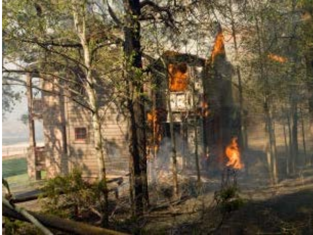
This home was lost because it had not proactively reduced risks posed by wildfire through homeowner action and hazardous fuels reduction before the Wallow Fire in Arizona, in 2011. Photo credit: Kari Greer.
