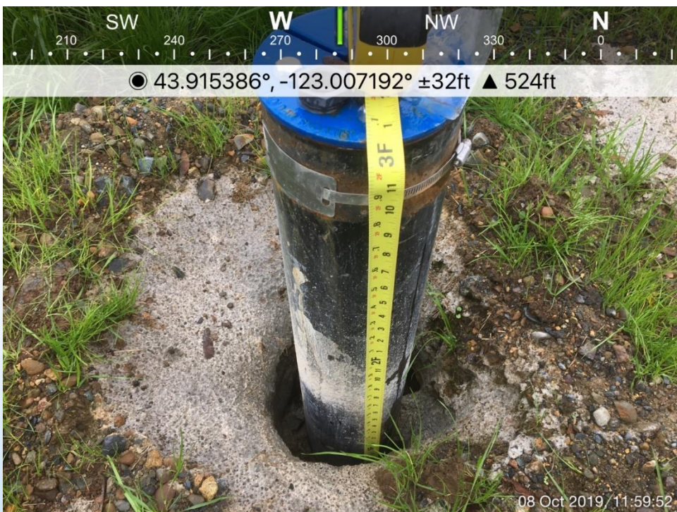
Improper seal
