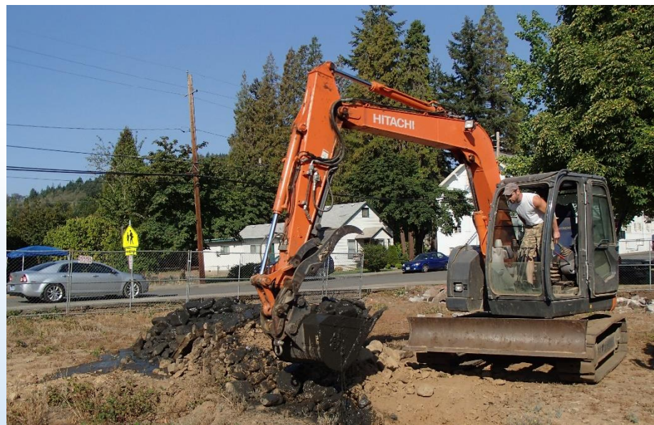
Abandonment of a dug well contaminated by oil
