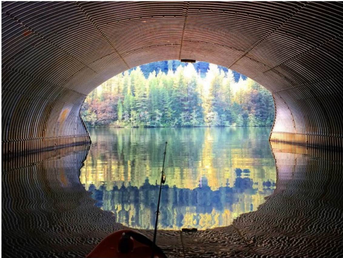
Culvert connecting North Fork Clackamas River to North Fork Reservoir, Linn, Oregon
