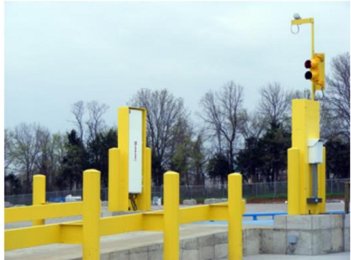
*Drive-Thru Radiation Detecting Portal Monitor*
