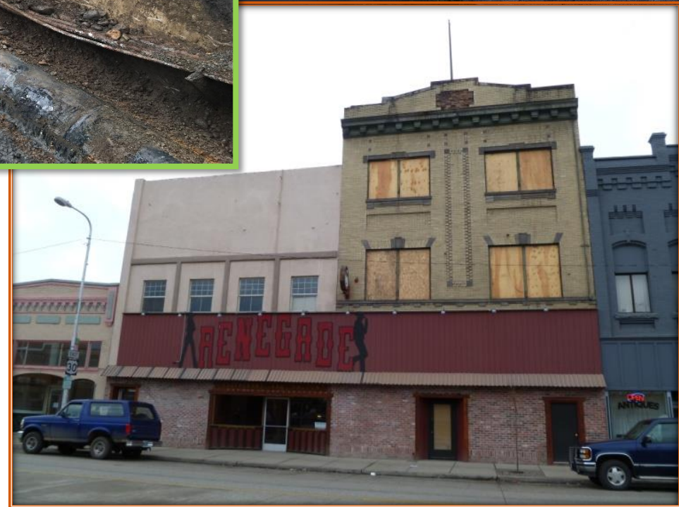
Staff Theater/Odd Fellows Building, La Grande
