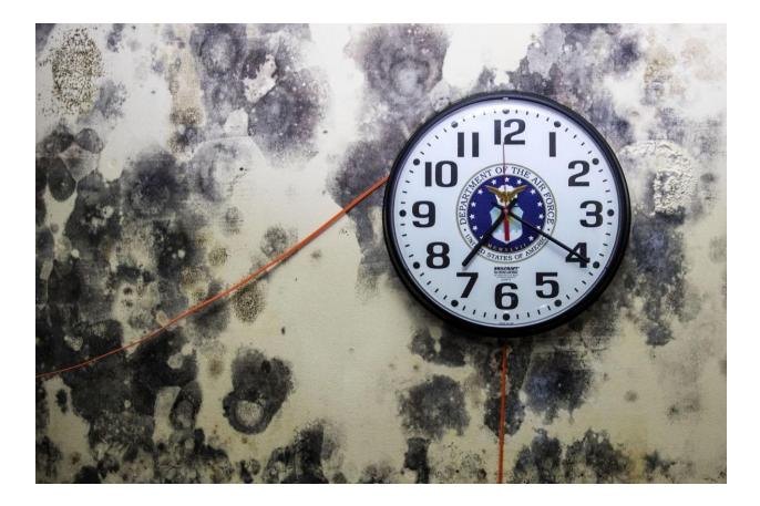
A stopped clock hangs on a mold-covered wall inside the 55th Wing headquarters at Offutt Air Force Base. The building has been abandoned and will be demolished after floods last March filled it with water 5 feet deep.
