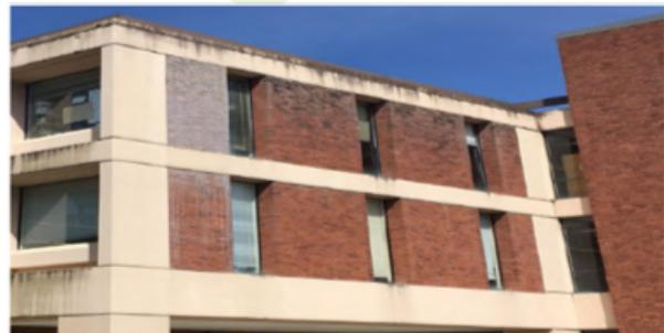
Evidence of efflorescence, water intrusion (parapet and walls) and poor thermal insulation (windows, in particular)
