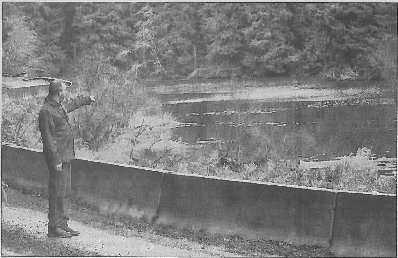
Newport Public Works Director Tim Gross indicates the site of the proposed new dam that would replace the existing high-hazard dams at Big Creek dams. (Photo by Cheri Brubaker)
