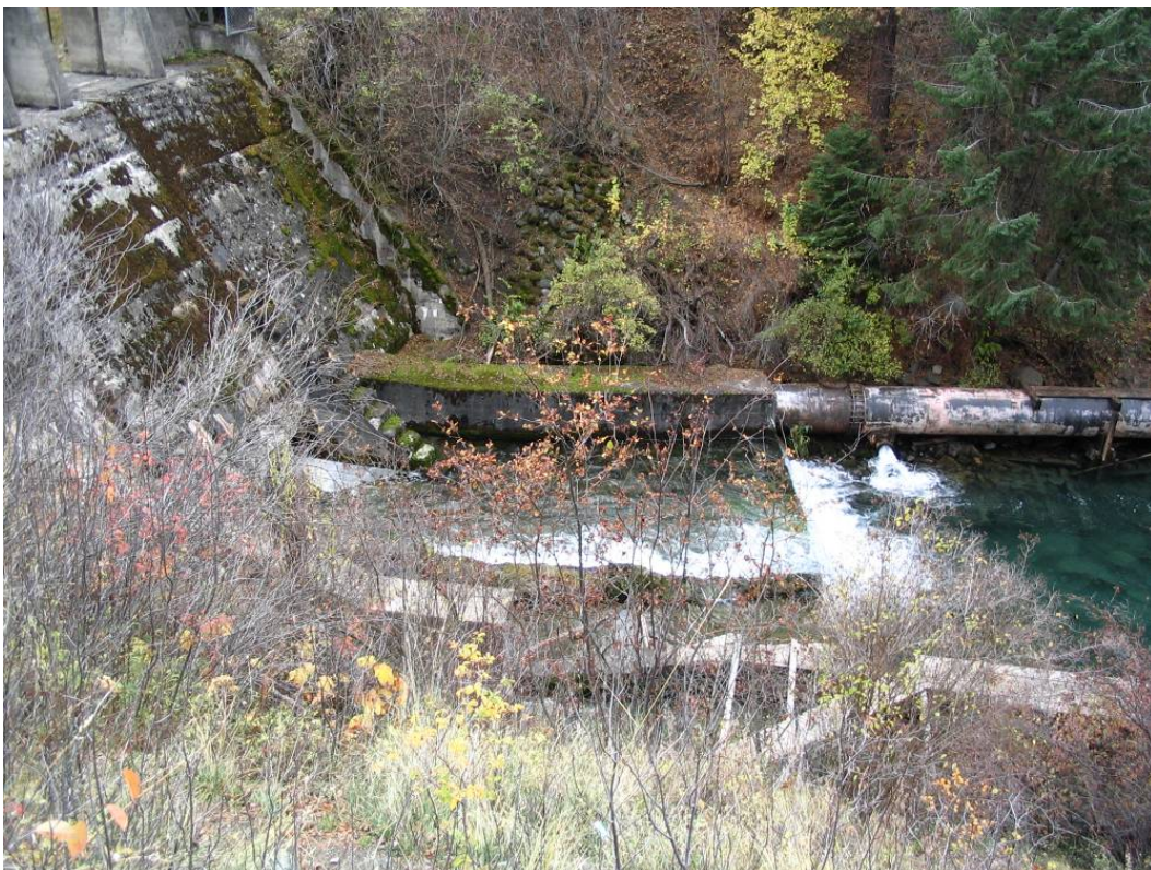
Photo 4. Downstream face of dam looking at the sill.
