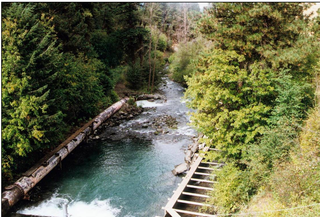
Photo 2. Looking downstream from the dam.
