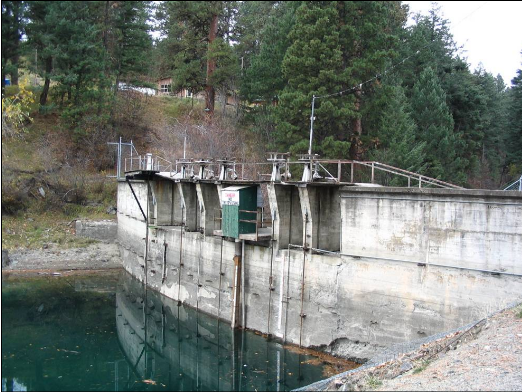
Photo 7. Upstream face of dam.
