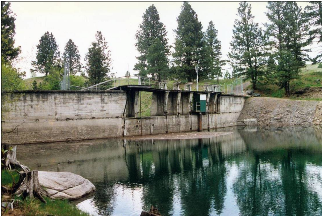
Photo 6. Upstream face of dam – 5 feet below full pool.
