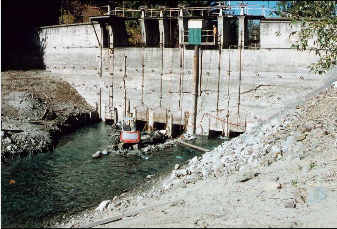
Photo 5. Upstream face of dam showing gates.
