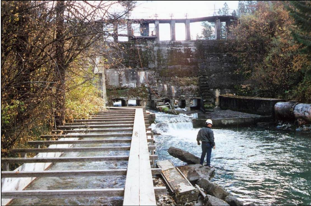
Photo 1. Downstream face of dam.
