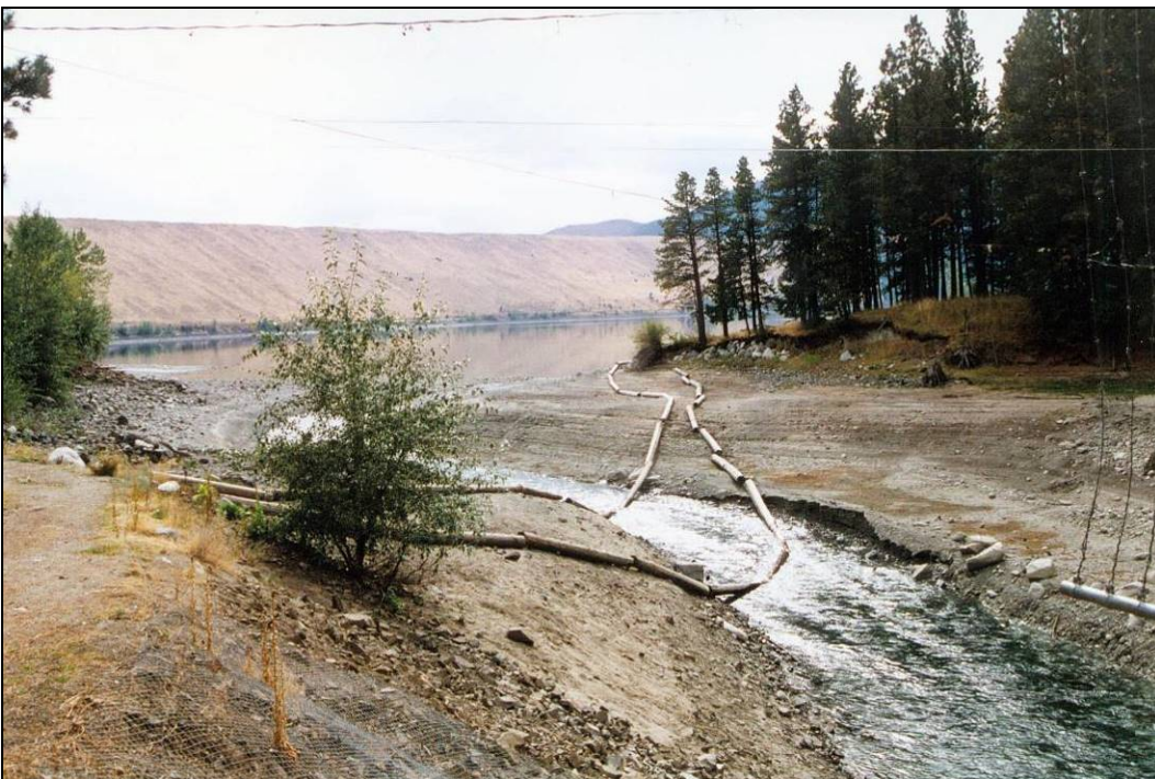
Photo 8. Looking upstream from the dam.
