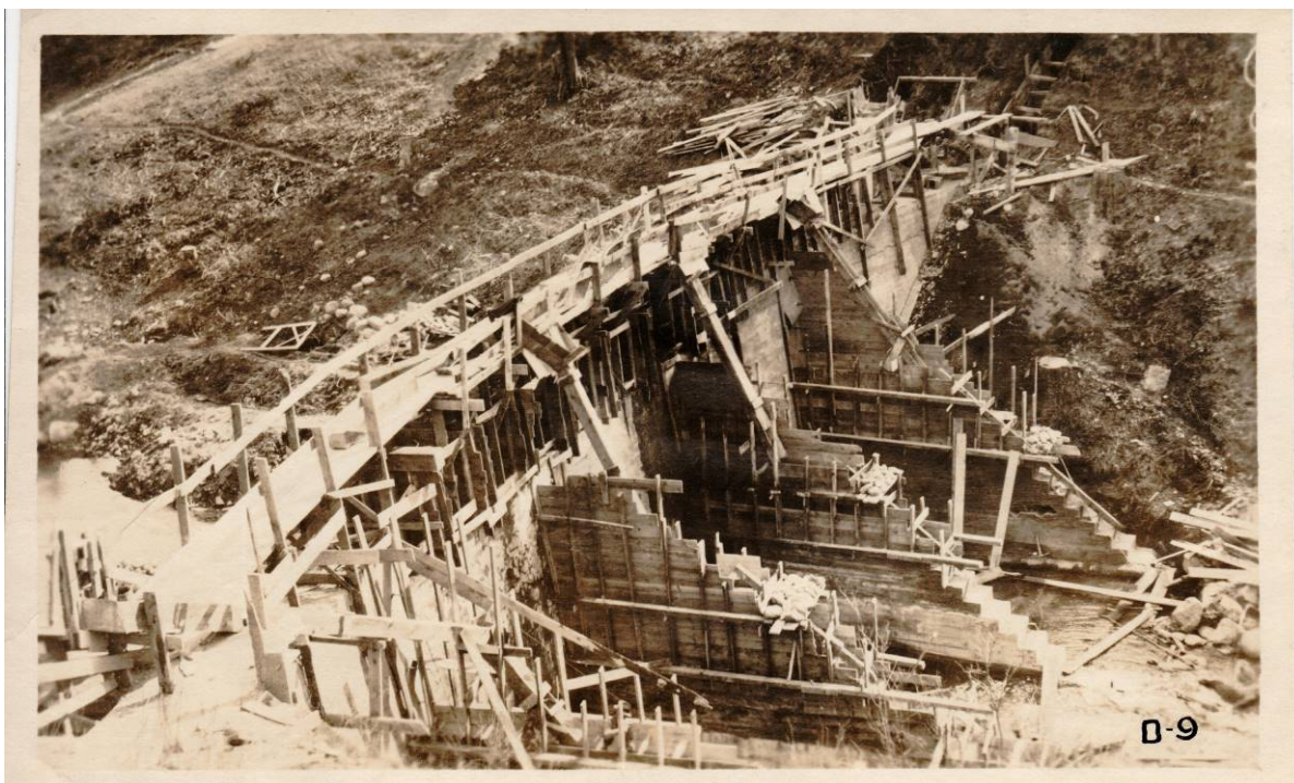
Photo 11. 1920 dam raise and adding downstream buttresses.
