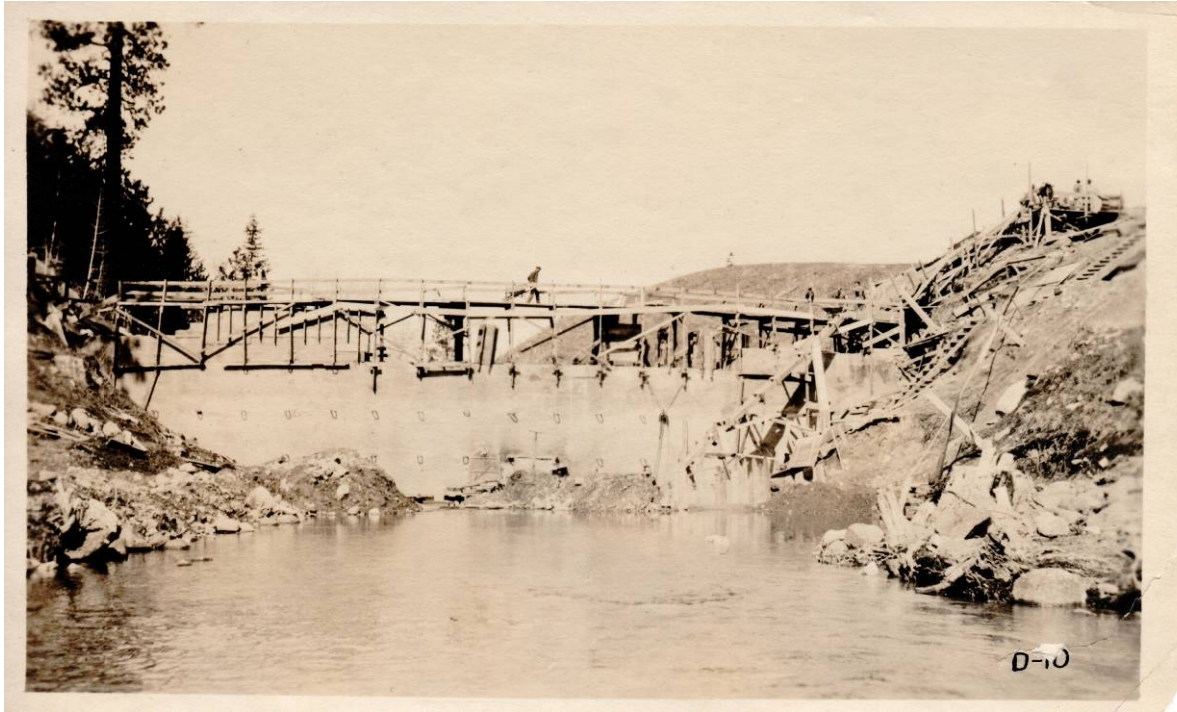
Photo 12. 1920 dam raise and adding downstream buttresses.
