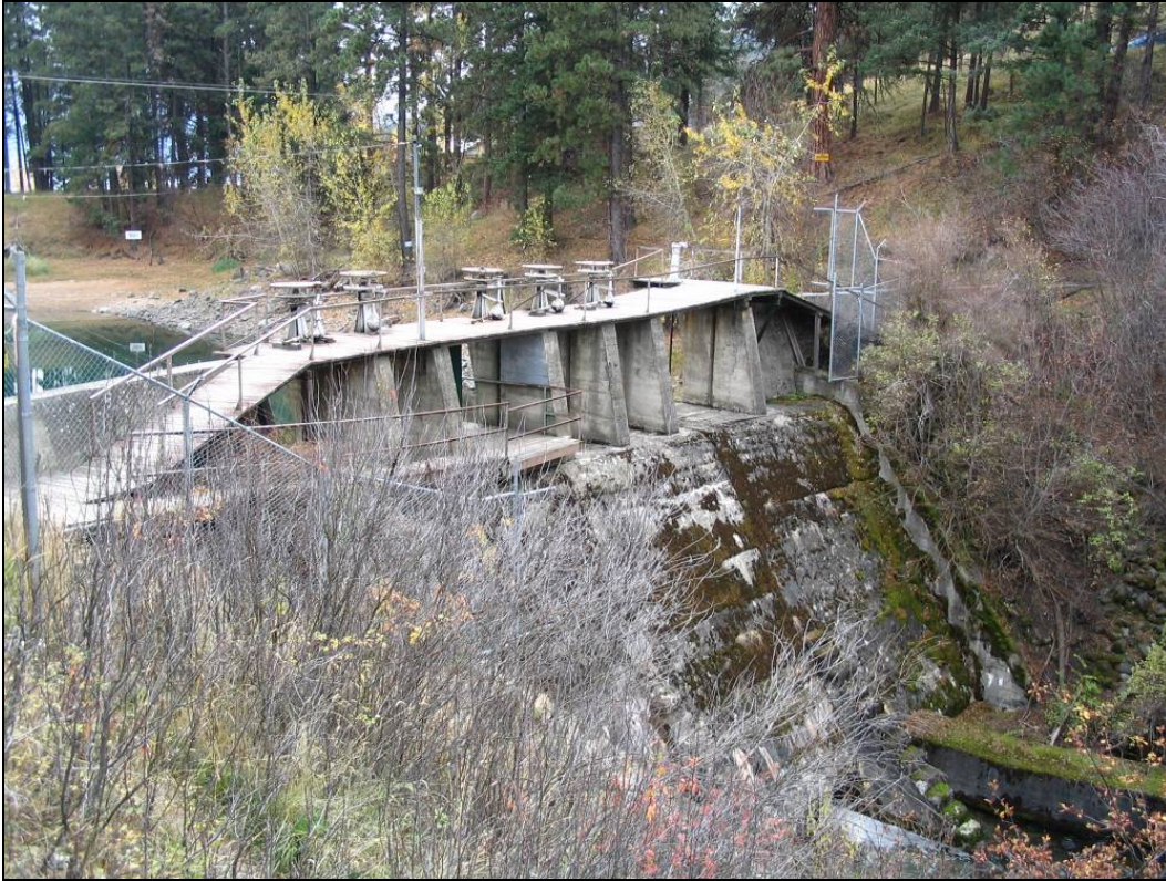
Photo 3. Downstream face of dam looking at the spillway.
