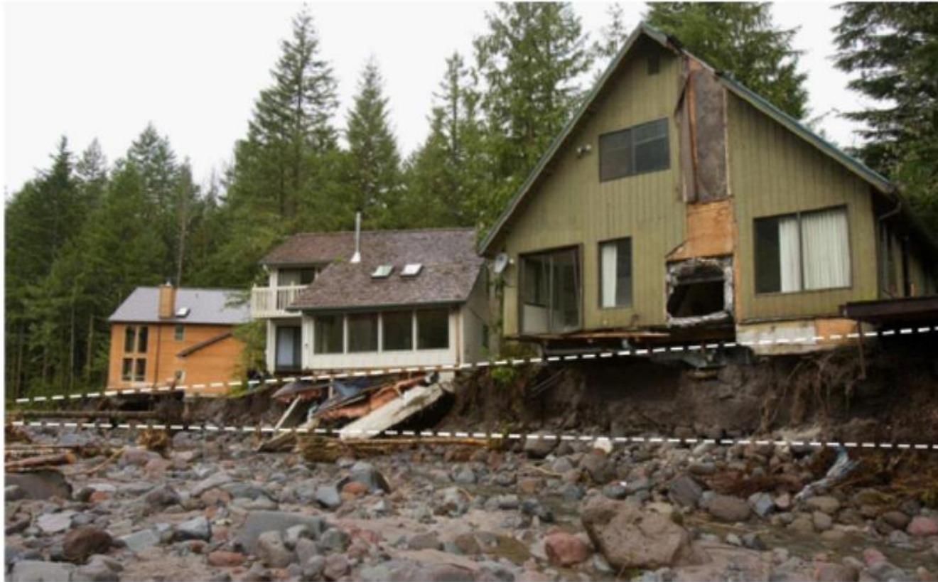
Damages resulting from January 16, 2011 flood, Zig Zag Village, Upper Sandy River
