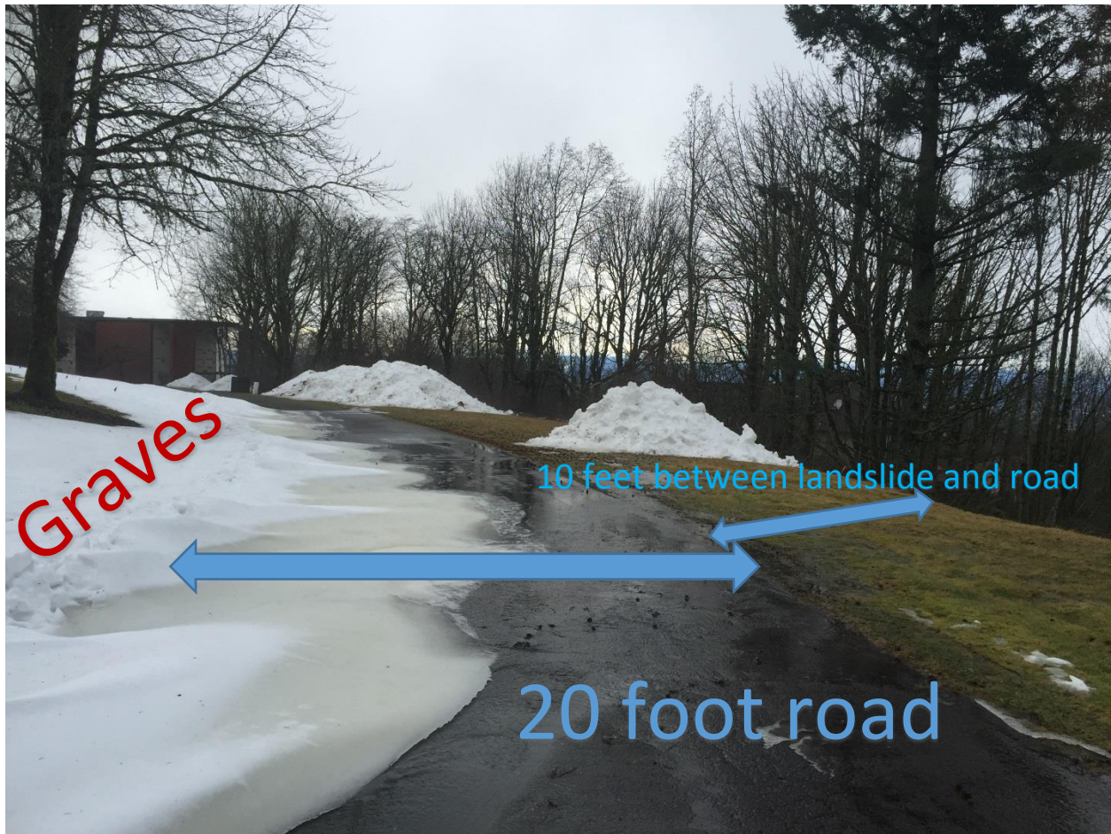
January 2017 Landslide at Skyline Memorial Gardens, Northwest Portland. Over 1,500 yards of earth
