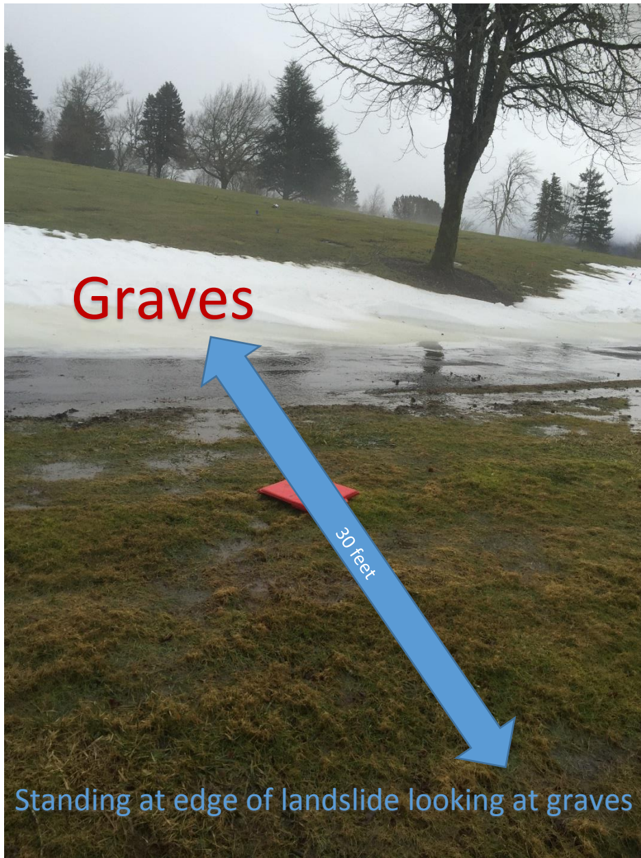
January 2017 Landslide at Skyline Memorial Gardens, Northwest Portland. Over 1,500 yards of earth
