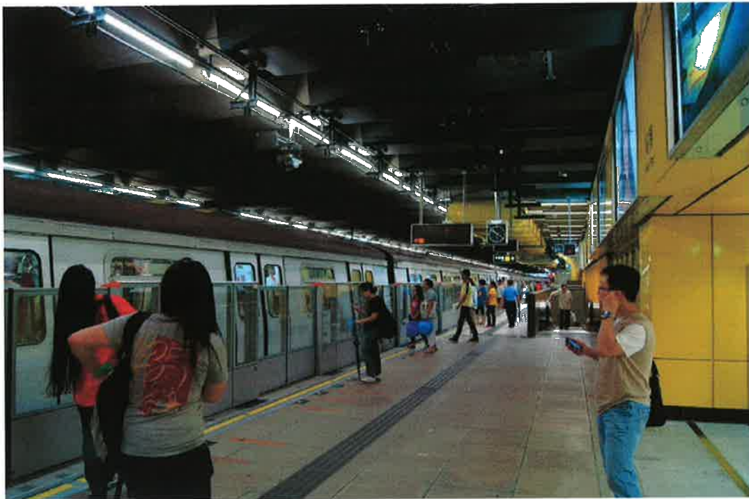
Figure 25. Platform edge doors at Kwai Hing Station of Hong Kong MTR. By Hokachung - Own work, CC BY 3.0, https://commons.wikimedia.org/w/index.php?curid=15843556
