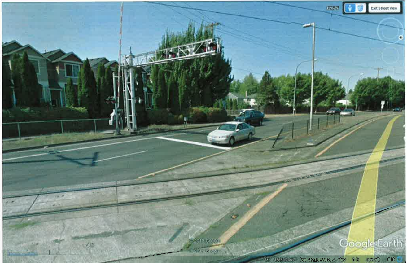
Figure 4. Deceptively safe crossing directs pedestrians into trackway when cars are stopped at crossing gates
