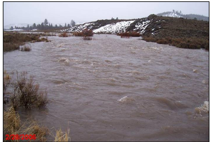
Figure 10: Alkali grade control structure on Last Chance Creek demonstrates the stability of the current design method during a flood in spring 2006. First photo is February 23, 2006, second photo taken on February 28, and third photo in May 2006. Note in the first and third photos that low flows remain in the constructed riffle-pool base flow channel after the flood. (Photos: Jim Wilcox)
