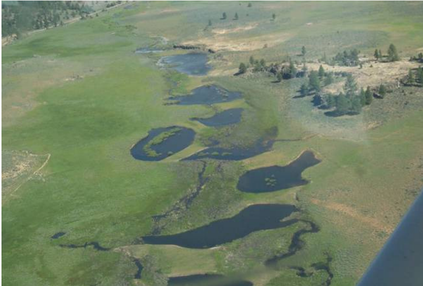
Figure 1: Post-project aerial photo of Last Chance Creek (2005). The series of ponds and plugs mark the location of the pre-project gully. The widths of constructed plugs indicate pre-project gully width. Historic remnant channels are used for the base flow channel of the restored system. (Photo: Jim Wilcox)
