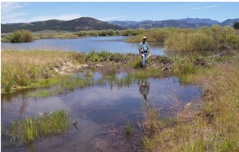
Figure 13: At the Red Clover - McReynolds Project, flow had cut through a plug shortly after construction due to damming of the designed base flow channel. Beaver subsequently dammed the cut at the plug so that base flow elevation is maintained upstream of the plug. (Photo: Joe Hoffman)
