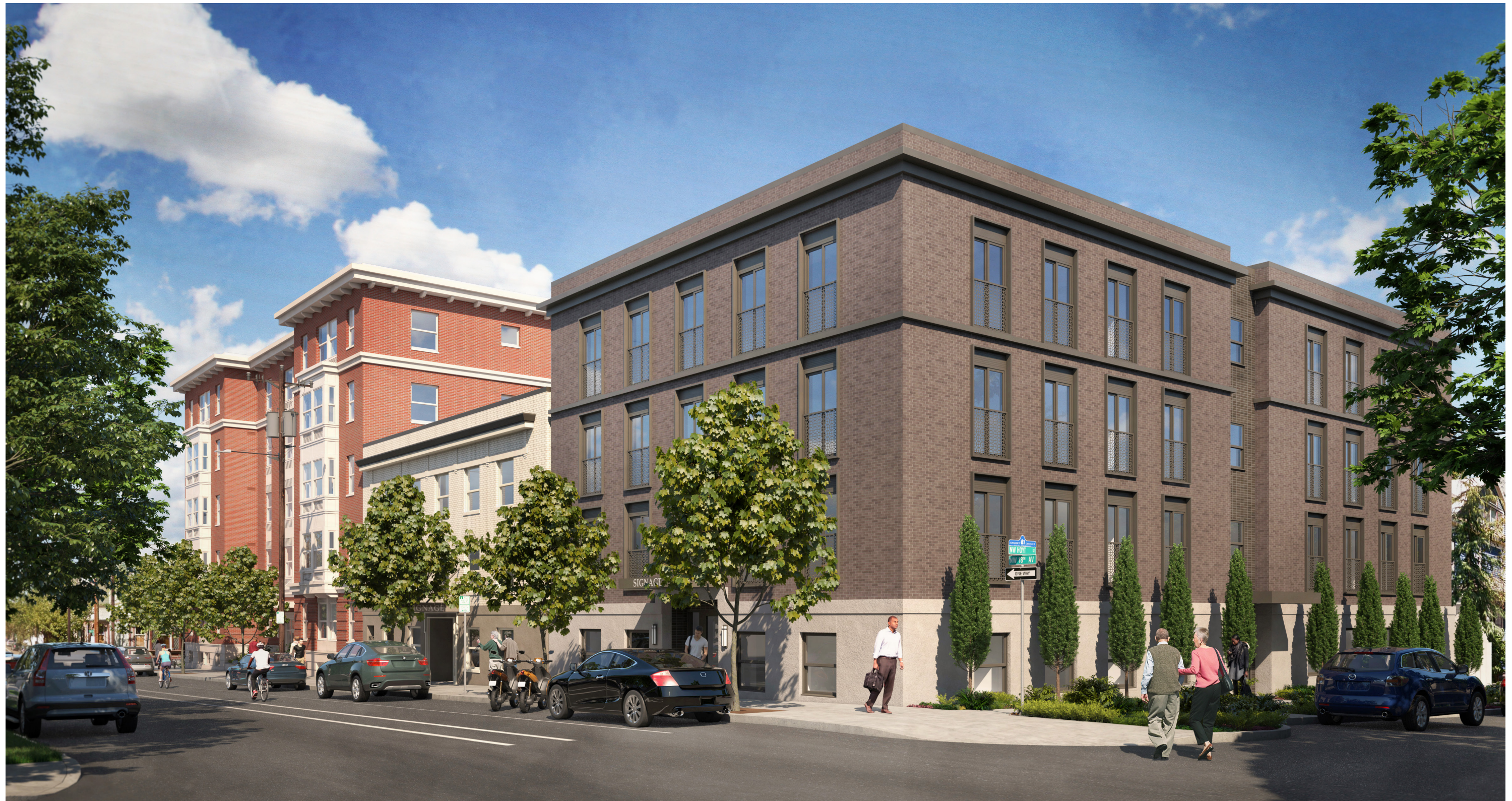
SW CORNER - NW 18TH AVENUE & HOYT STREET
