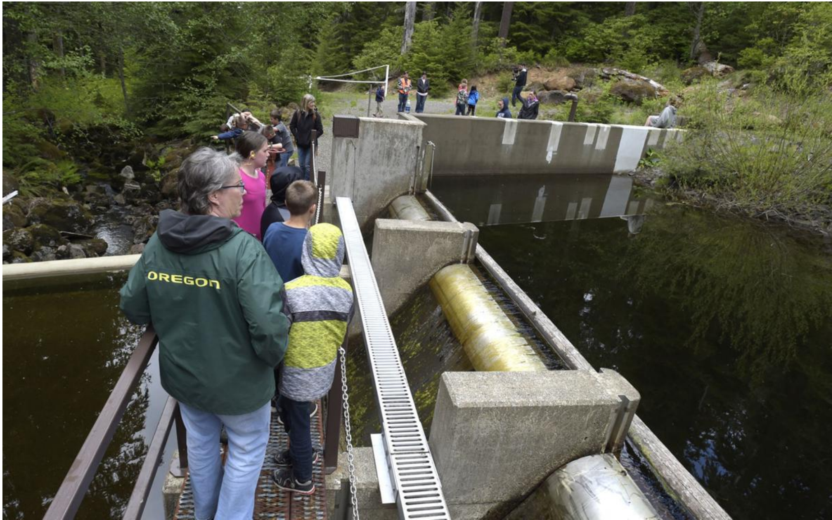
At the top of the mountain is the intake structure where it all starts
