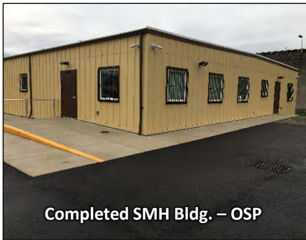
SMH Treatment Building Construction - OSP
