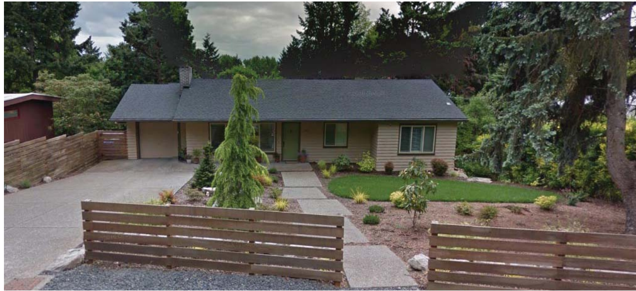
PHOTO Existing House
