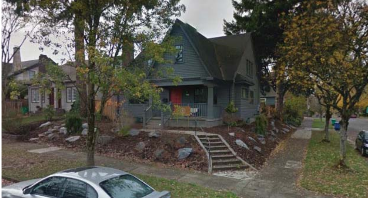
PHOTO Existing House
