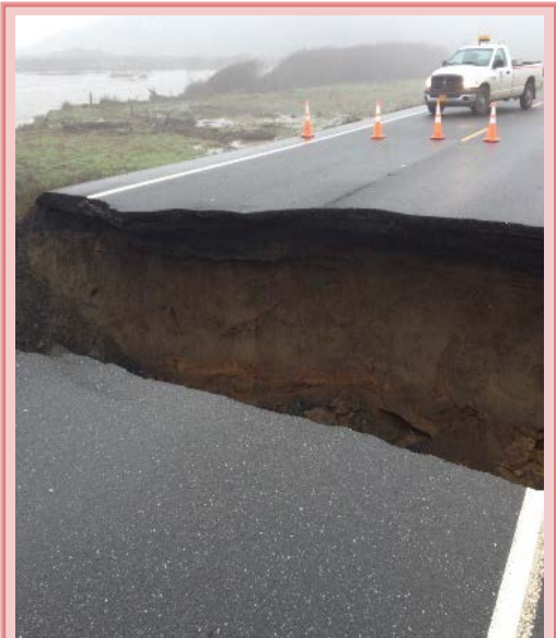
Culvert failure on U.S. 101 along the south coast (Dec 2014).
