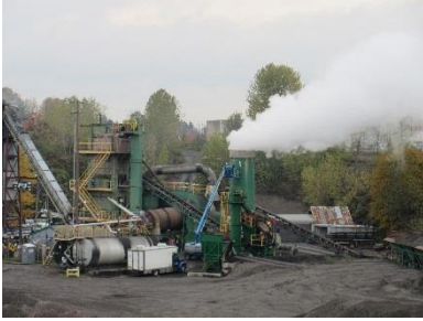
State-of-the-art pollution and odor control technology at a batch asphalt plant.
