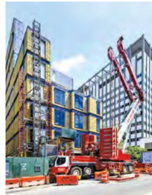
While the Carmel Place modules were under construction at the Brooklyn Navy Yard, the building's foundation and ground floor were being prepared on East 27th Street. The modules were assembled in just four weeks, greatly reducing construction noise and disruptions to the building's Manhattan neighbors.
