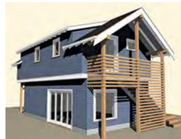
The ADU entrance stairway is accessed through the side yard, behind a slatted cedar screen wall. This feature acts as a guardrail and hides mechanical equipment, including an energy-saving tankless gas water heater and HVAC heat pump.
