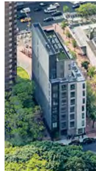
The Carmel Place building is composed of four staggered, 11-foot-wide towers, each corresponding to a column of stacked modules. Bricks in four shades of gray were chosen for the facade.
