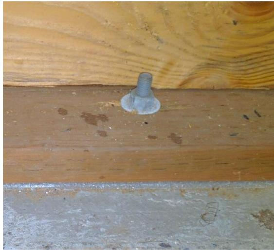
A home that is not properly bolted to its foundation could slide off of it during a CSZ earthquake, making it unsafe for occupation
