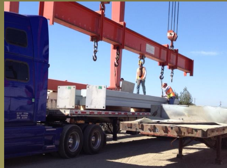
Column Fabrication – Steel Rebar Reinforced, Pre-cast, Wall Support Columns
