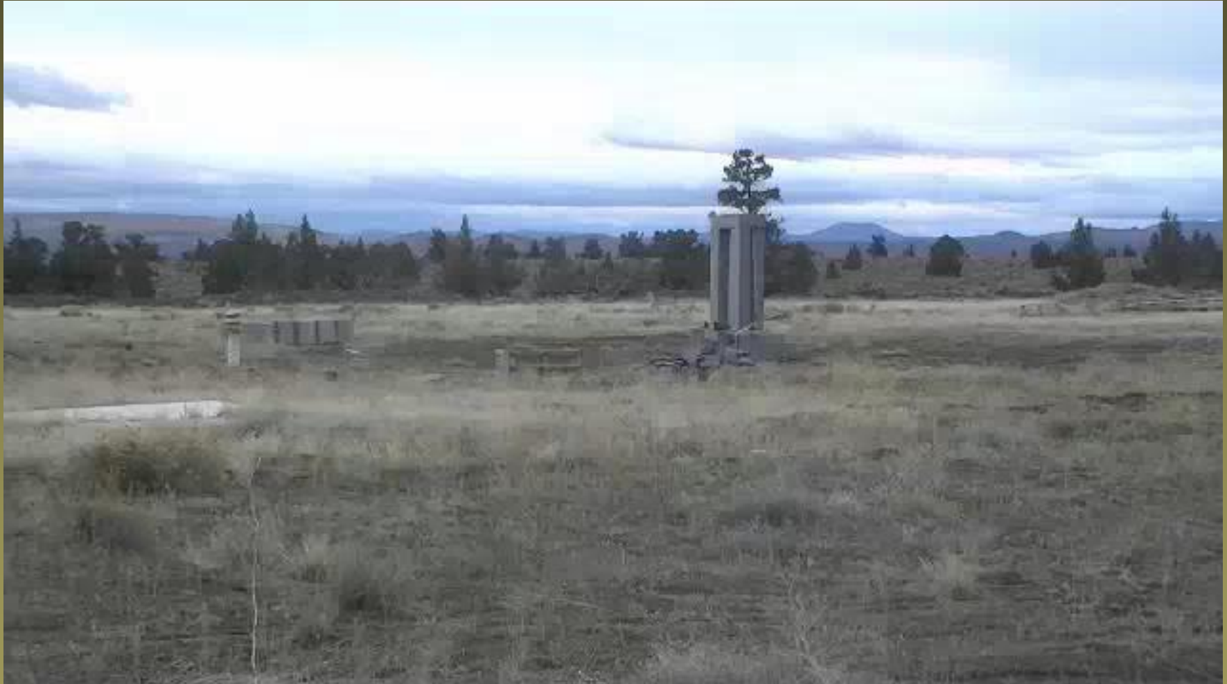
Recent Wall Design - Blast Verification Test
