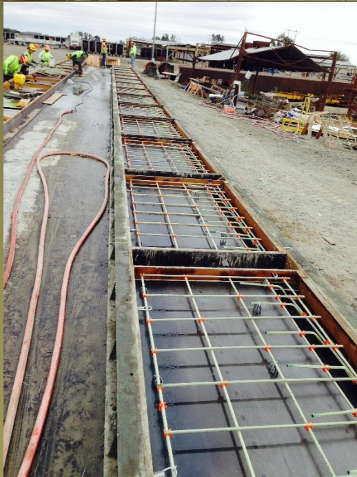
Wall Fabrication – Composite Rebar Reinforced, Pre-cast Transformer Protection Walls
