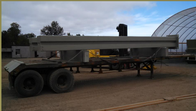
Column Fabrication – Steel Rebar Reinforced, Pre-cast, Wall Support Columns
