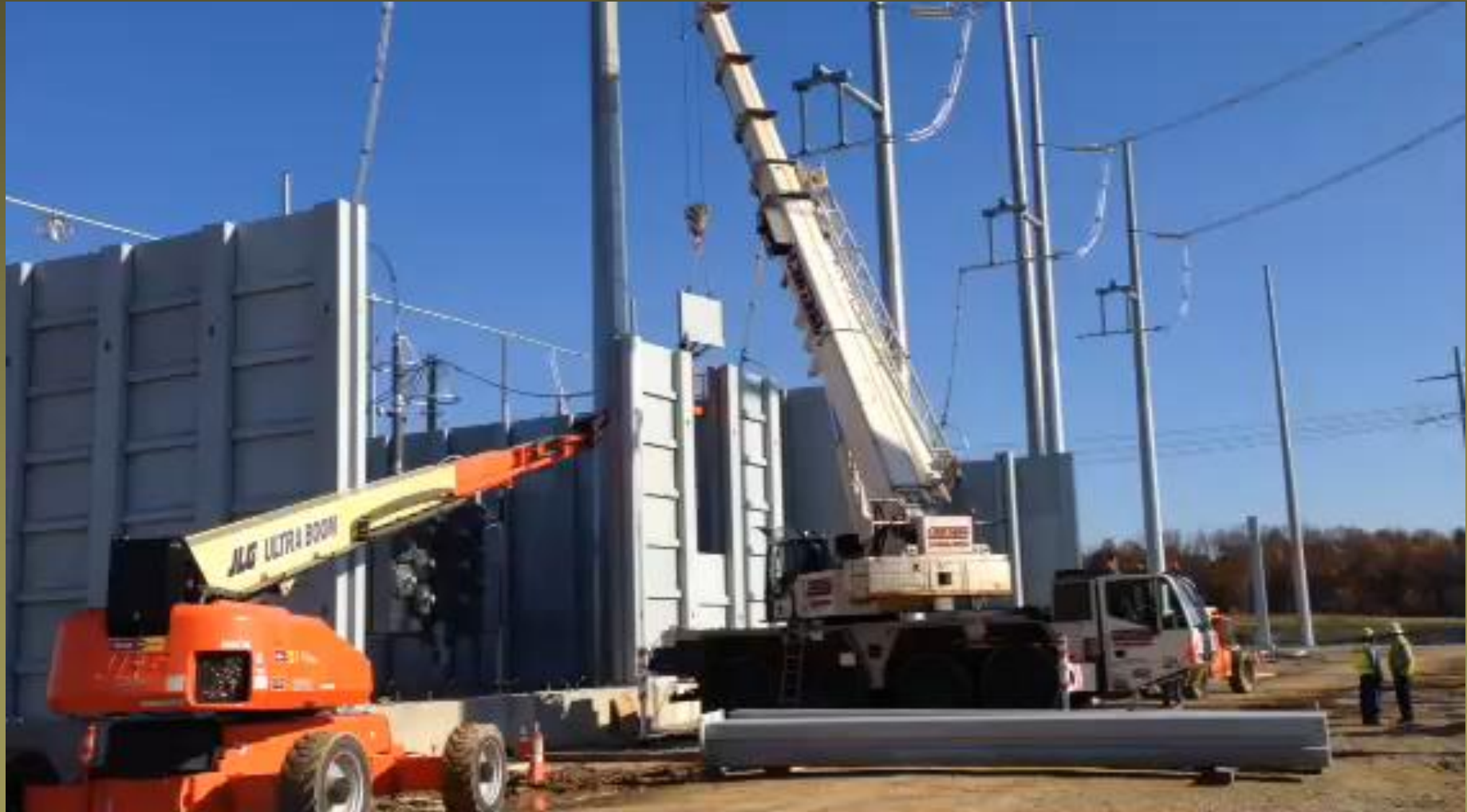
Wall Installation – Composite Rebar Reinforced, Pre-cast Transformer Protection Walls
