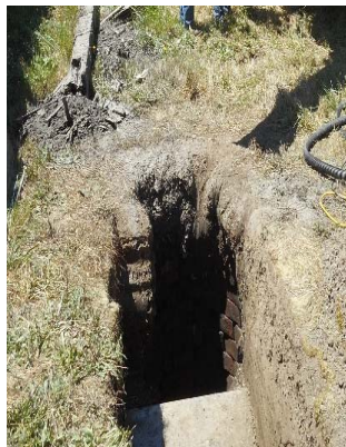
Hand dug well abandoned in Lafayette, Oregon
