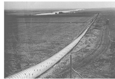
Circular irrigation flume for the Goose Lake Valley Irrigation Company in Lake County, Oregon, 1915 (Photo from Salem Public Library Historic Photograph Collections, Salem, Oregon; Oregon State Archives, Secretary of State, OWR0152)
