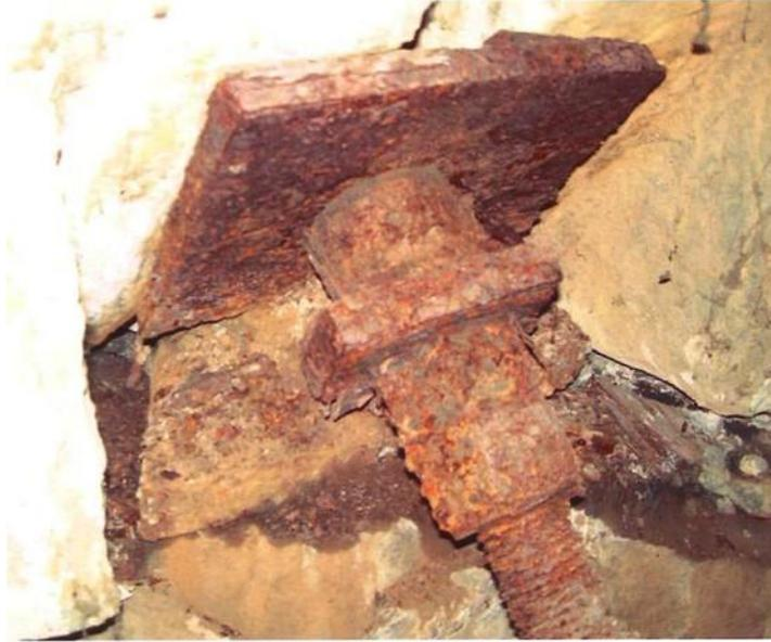
Severely corroded surface-mounted gudgeon anchor.
