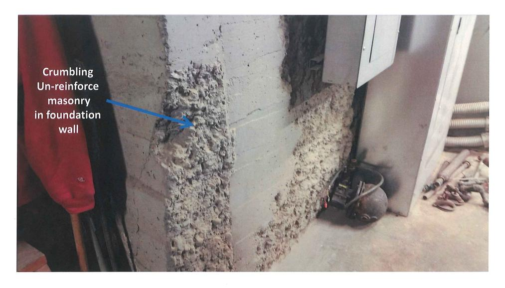
Foundation Wall of un-reinforced masonry of courthouse You can see partly why we were ranked  $4^{th}$  worst in the state here
