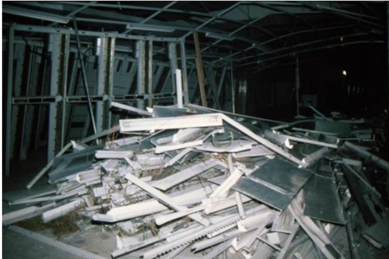
**Picture 2** – The overhead lighting fixtures in a Central Office failed during an earthquake. Note the equipment in the background was supported by “jiffy poles” after the earthquake. Mexico City, 1985.
