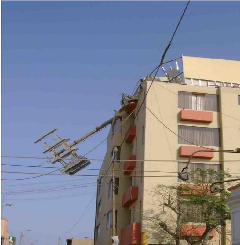
*Cellular Base Station tower failure, this site is installed on roof of an apartment building, which is not designed for critical infrastructure facility. Pisco, Peru earthquake 2007*
