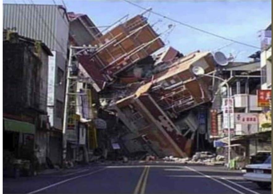
*Cell site collapsed with the commercial building collapse. Chi Chi earthquake Taiwan, 1999.*
