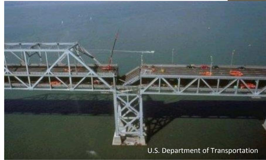
*San Francisco - Oakland Bay Bridge after the 1989 Loma Prieta earthquake. An example of bridge failures that could impact utility conduits supported by or integrated into the bridge.*
