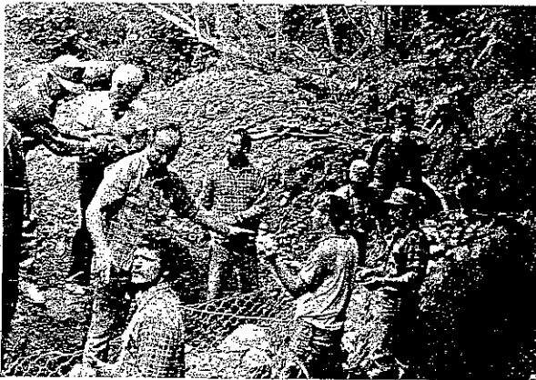
Volunteers fill the gabions by hand with rock donated for the project.
