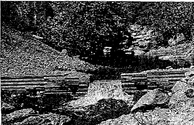
A wooden sill used to collect spawning gravel.
