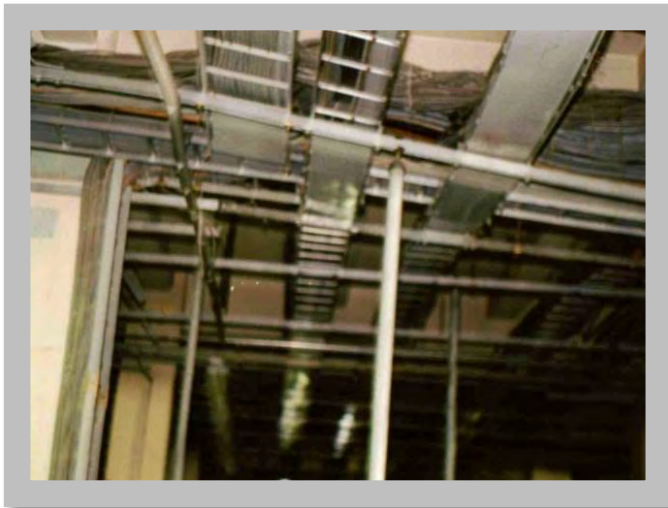
Figure 7.13: Super structure of cable racks failed due to lack of detailing and in many cases, overload. Whittier Narrow earthquake, California, 1987. (Source: Alex Tang)
