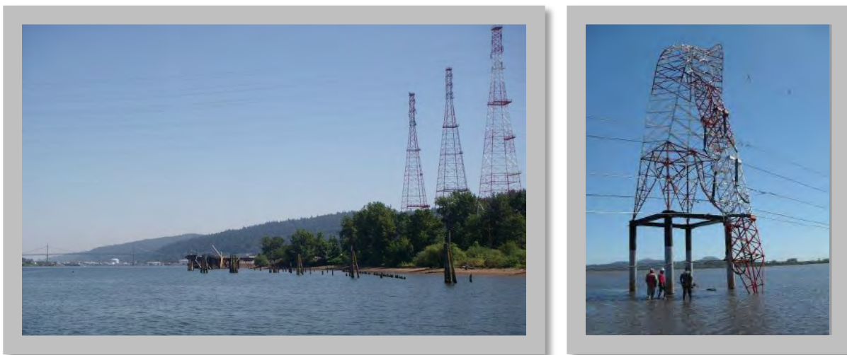
Left: These high voltage electrical transmission towers are built on a river bank in the Critical Energy Infrastructure (CEI) Hub susceptible to lateral spreading. (DOGAMI photo) Right: Structural damage to a high voltage transmission tower located at a river crossing in 2010 Chile earthquake (ASCE Technical Council on Lifeline Earthquake Engineering – TCLEE)
